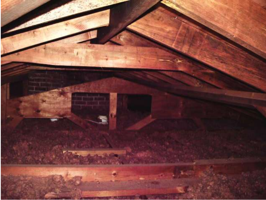
Bonus pic: Girder truss used to support ceiling at family room.
